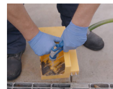
STEP 6 Clean drain saver
