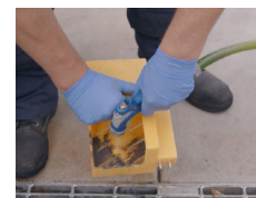
STEP 6 Clean drain saver
