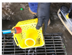
STEP 8 Empty and clean drain saver
