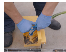
STEP 6 Clean drain saver
